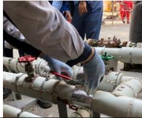
Carefully position tape on joint, cut it into the length accordingly.
