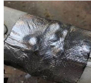
Installation done. No wrinkles over the time.
